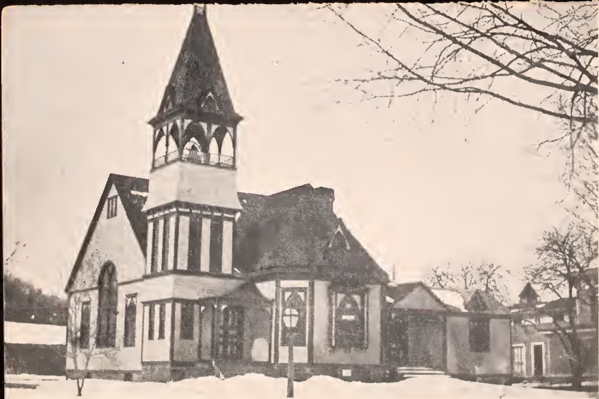
BERKSHIRE, N. Y. Methodist Episcopal Church.
